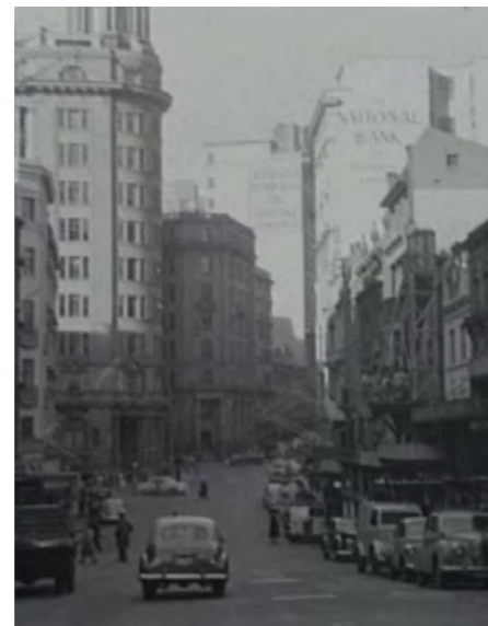
30. View looking East along Hunter st, 1954. Subject Eastern Metro site is situated.
