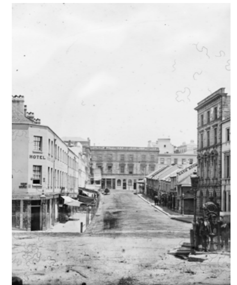
34. View looking west along Hunter St near corner of Pitt and O'Connell st, 1870-75.
